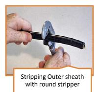
Fig 2.3.21: Splicing preparation
